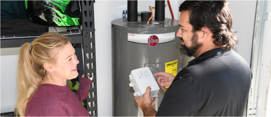
Pictured above: CHELCO Energy Advisor Tyler (right) speaks to a member about the load control switch before it is installed.
