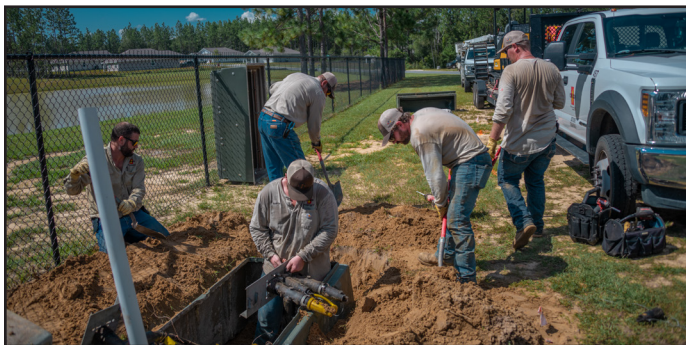
A CHELCO line crew works on underground equipment.
